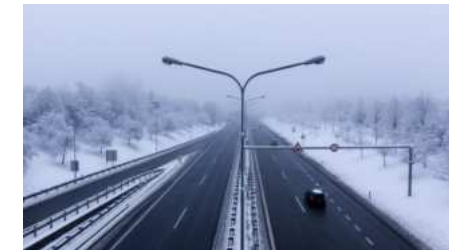
Czech Republic Road weather national system
